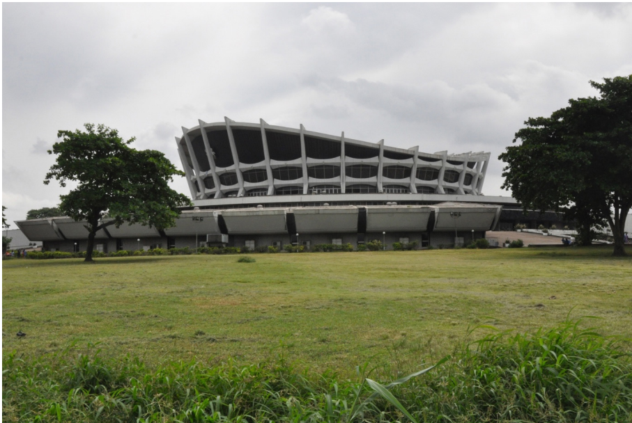
Image 2 National Theatre, Lagos, Nigeria. S. Kolchev (design architect) for Technoexportstroy (Bulgaria), 1977, photo Ł. Stanek, 2015
