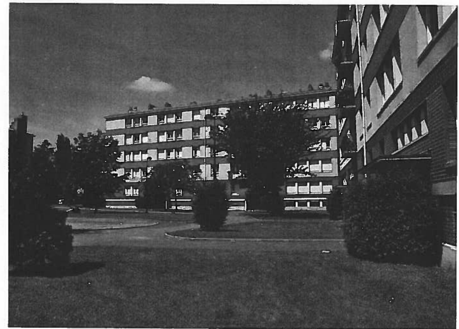
Figure 6.2 Robert Auzelle, Cité de la Plaine in Clamart, collective housing estates, current state, photographed by Łukasz Stanek in July 2012.
